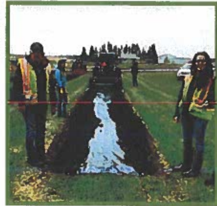
Rebekah Adams of AWES (right), Terry Stefiuk of Town of Two Hills (left) and other town and County staff laying the mulch blanket for the Eco-Buffer.
